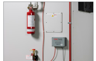
Fire Suppression System
